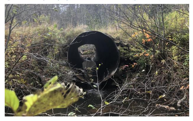
Figure 36: Complete barrier to fish passage on north branch of reach 6 - MacKinnons Rd (61°17′33.3″W, 45°57′3.4″N).
