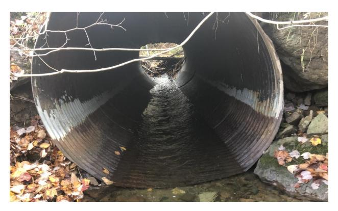
Figure 35: Partial-to-complete fish passage barrier on reach 6 MacKinnon Rd crossing (61°17′38.2″W, 45°56′60″N).
